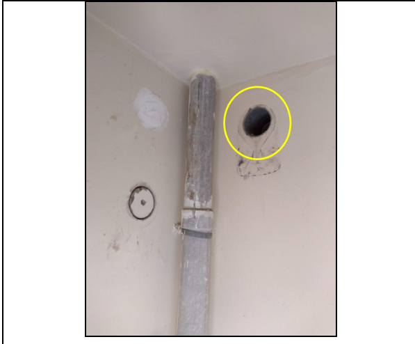
3. Compartmentation break to incinerator cupboard (6 th floor).
