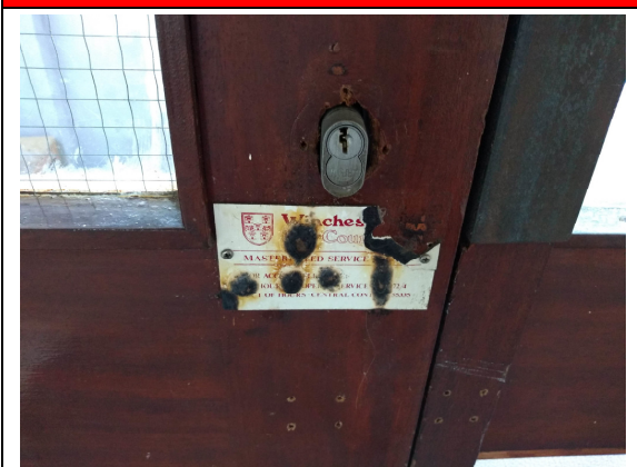
11. Vandalism to 8 th fl landing door.
