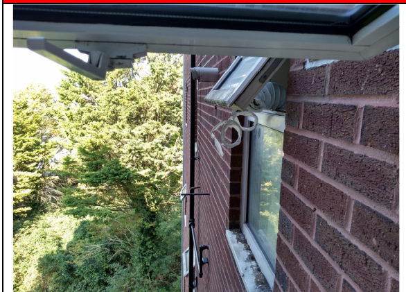
17. Tumble dryer hose vent to flat.
