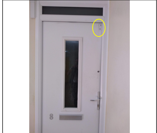
10. Damage/ repair to flat 8 door.
