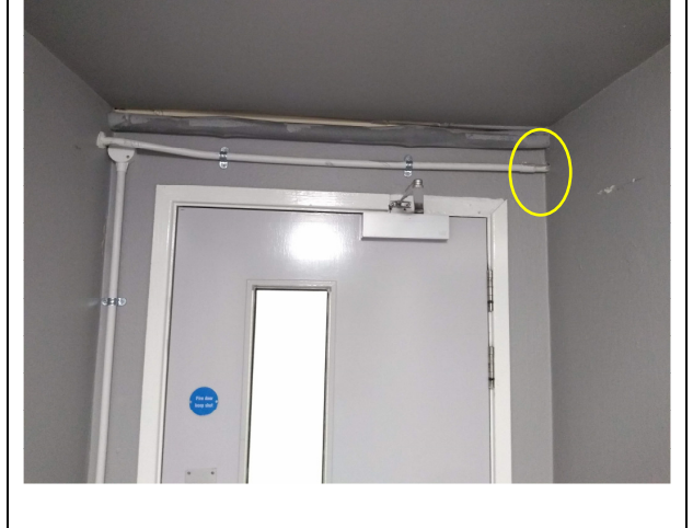
2. Fire stopping missing to conduit.
