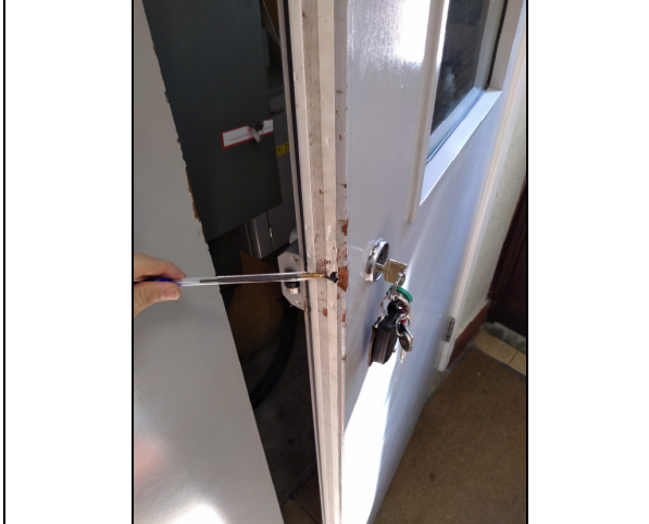
1. Damaged smoke seal to FD30.
