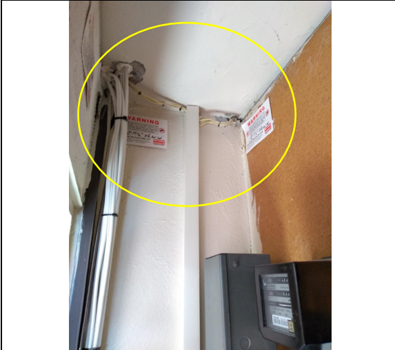
9. Fire stopping to service cupboard.
