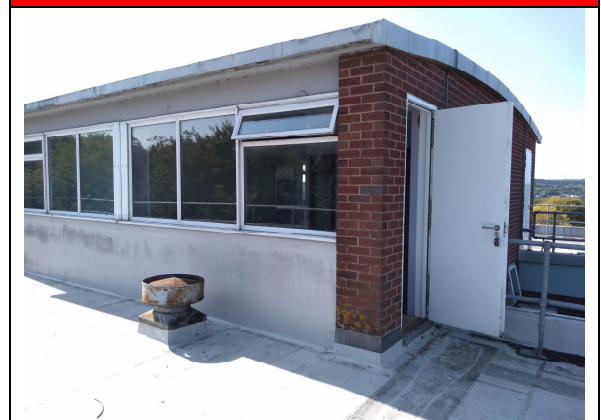
12. 8 th floor structure & roof.
