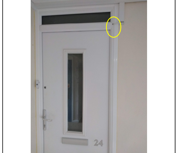
16. Flat 24 hole to doorframe.
