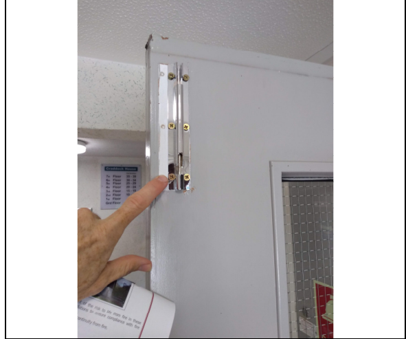
2. Bolt to FD30 broken, service cupbd.
