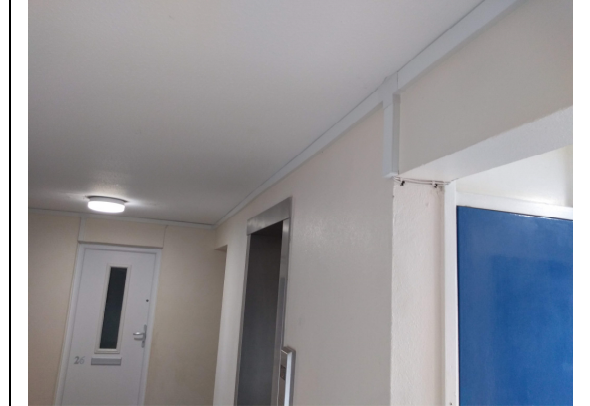
10. Cabling conduit to landing.
