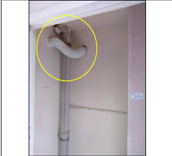
3. Compartmentation break to incinerator cupboard (5 th floor).
