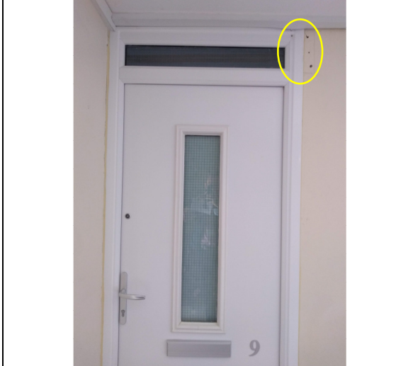
15. Flat 9 hole to door frame.
