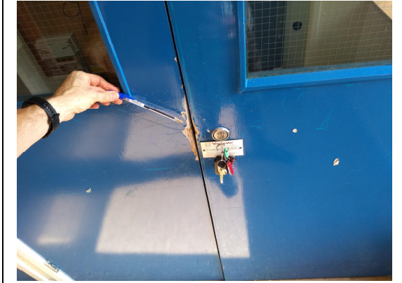
9. Damage to cupboard doors.
