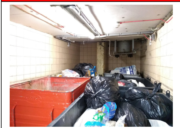
5. Bin store & sprinkler system.
