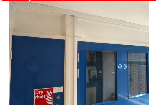
8. Loose telecoms cables to service cupboard .
