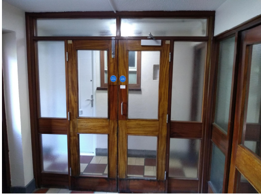
1. Double fire-doors to corridor.
