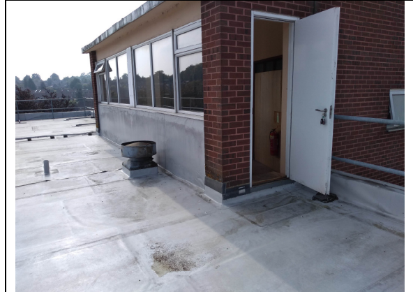
10. Roof & lift motor room structure.
