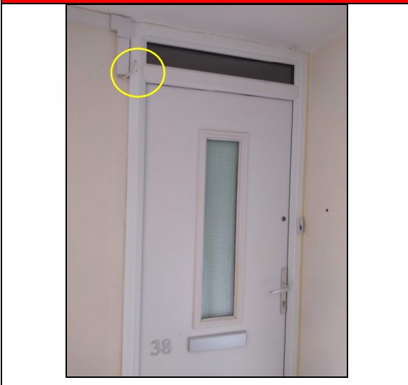
11. Flat 38: hole to door-frame.
