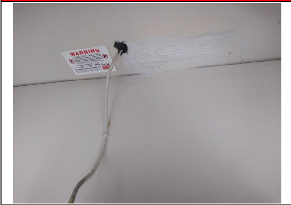
7. Fire stopping to service cupboard.
