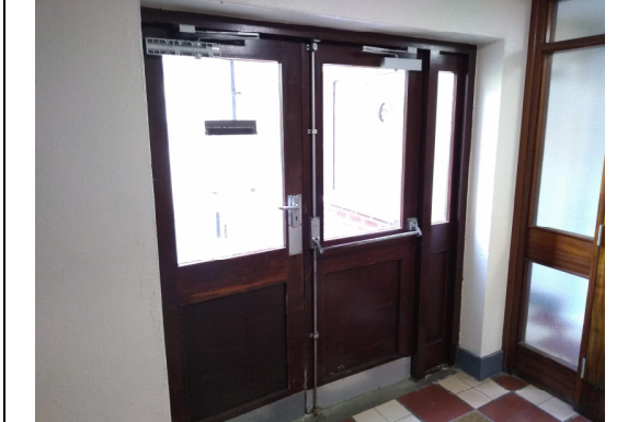
3. Escape doors to gr. fl. of stairwell.
