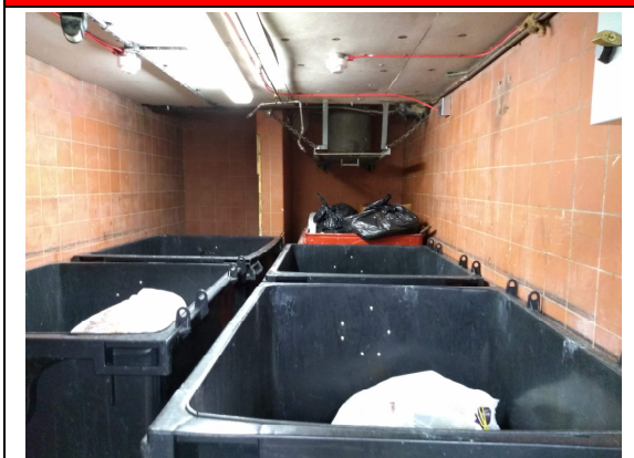
5. Bin store & sprinkler system.
