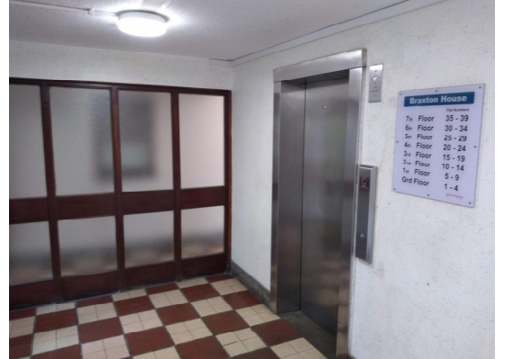
2. Lift lobby and glazed screen.
