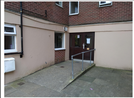
9. Rear exit & gas pipework.
