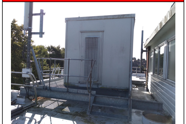
12. Telecoms shed on roof.
