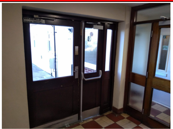
6. Escape doors to stairwell.
