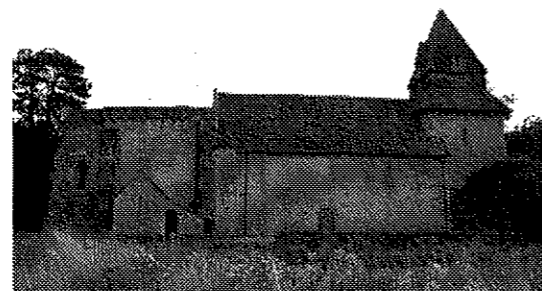
NORTH ELEVATION Photograph 5
