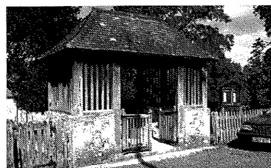
LYCH GATE Photograph 7
