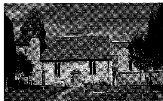
SOUTH ELEVATION Photograph 6
