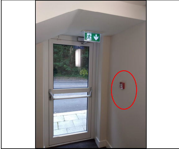
7. Escape door, ground floor.
