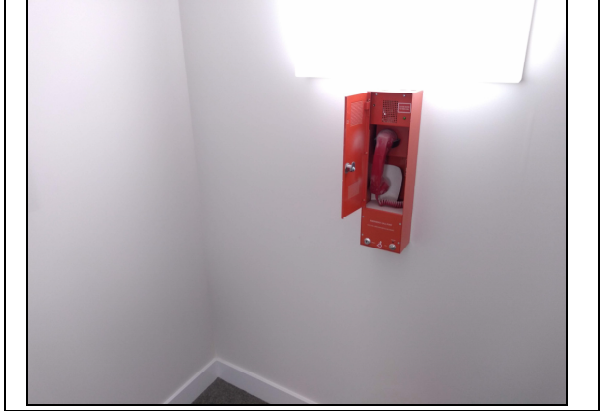
2. Refuge intercom box opened.
