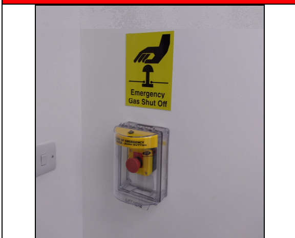
11. Gas shut off to laundry room.
