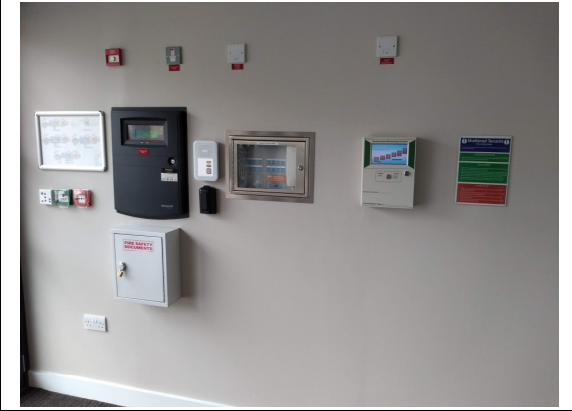
1. Alarm Panels in reception area.
