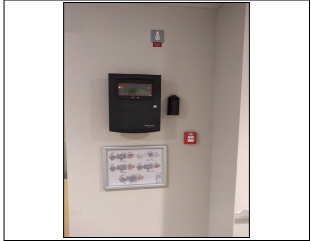
8. Alarm repeater panel.
