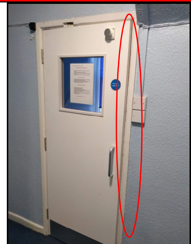
6. Fire-door not fully closing.
