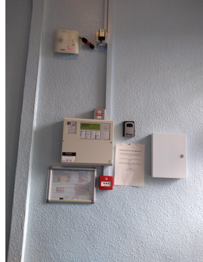
2. Fire alarm panel & tunstall.
