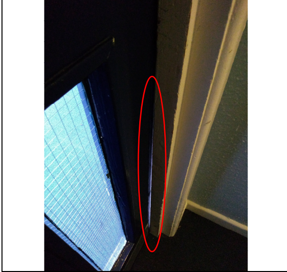
7. Gap at fire-door door stop.
