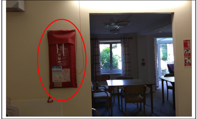
4. Fire blanket to the kitchen – recommended for replacement.
