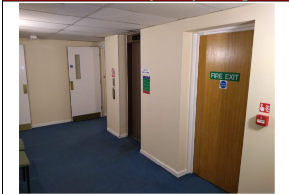
9. 2 nd floor lift lobby: call point sign.
