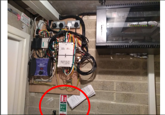
3. Lobby to lift motor room: CO 2 extinguisher missing.
