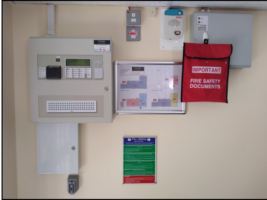
1. Fire alarm panel in lobby.
