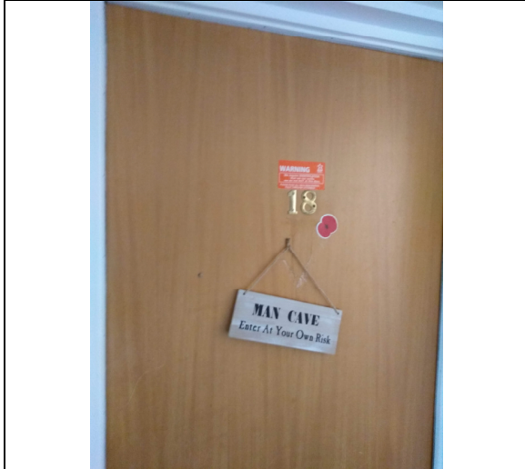
7. Flat 18 door: hook nailed to door.
