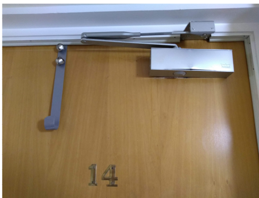
5. Damage to door closer of flat 14.
