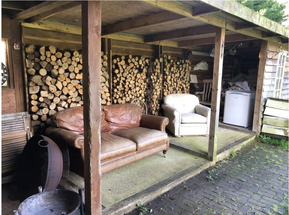
The extension to the stable block was erected in May 2011.
