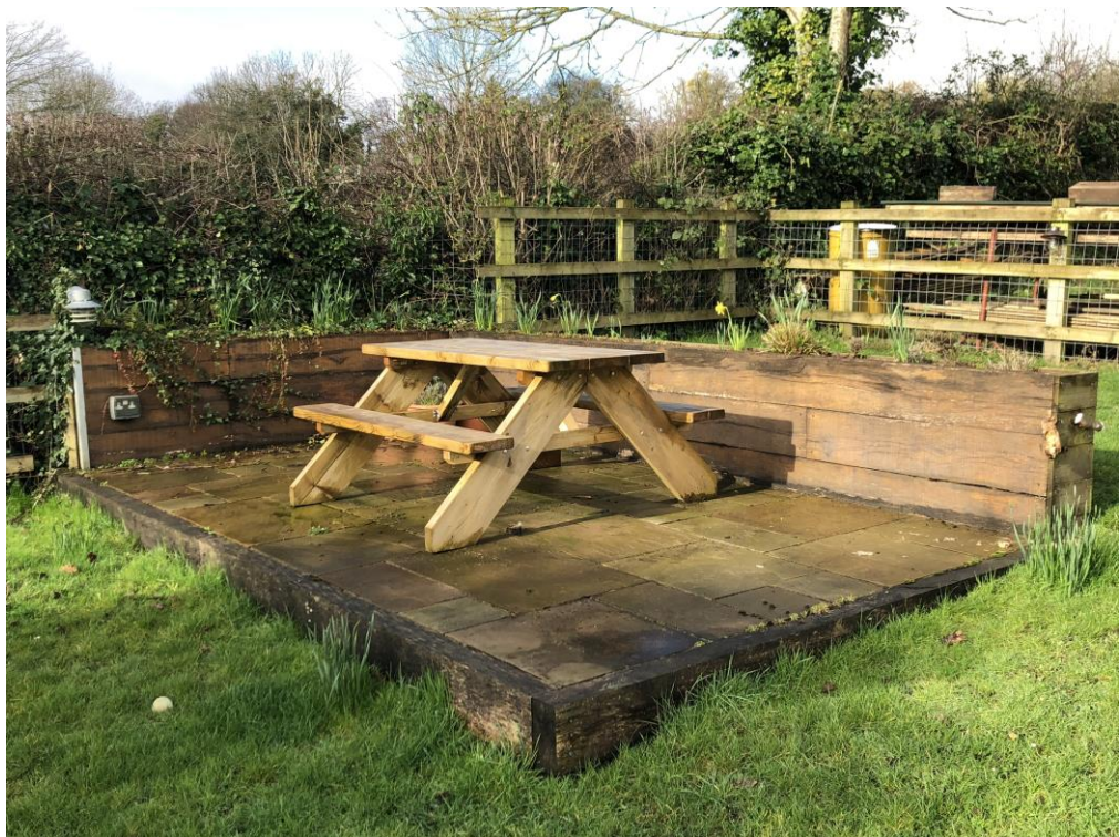
The patio was laid between May 2014 and June 2015.
