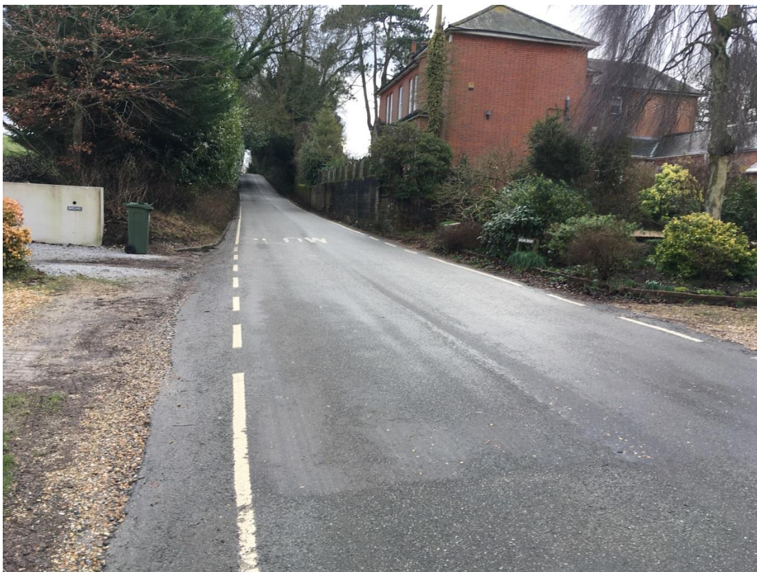
Photograph 2 – Main Road to the south-east
