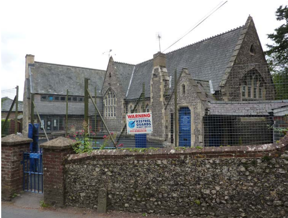
Figure 25: The Village School , Church Lane, of 1852-3, sits close to the church and is also built in a Gothic style. The high wire fence and warning signs degrade the setting of the listed building and represent a significant visual intrusion into the Conservation Area. Their removal would be welcome.
