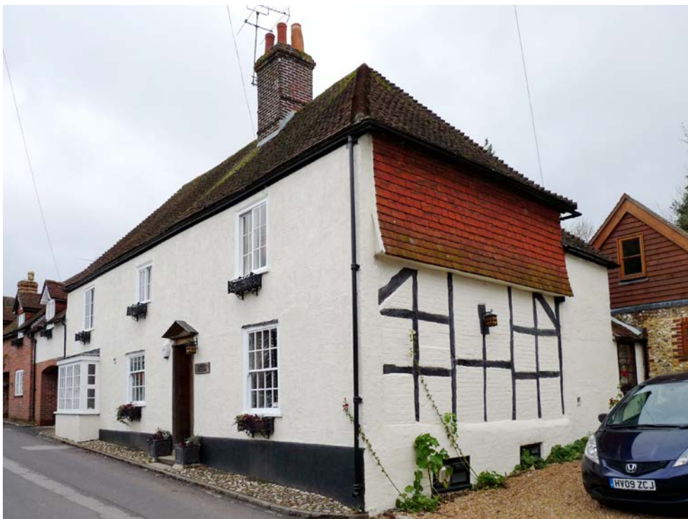
Figure 38: The Baechus , East Meon Road. An early 19 th century brick facade hides a 17 th century or earlier timber frame which is still exposed on the gable end.
