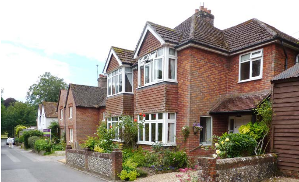
Figure 45: Later 19 th and 20 th century houses in Doctors Lane
