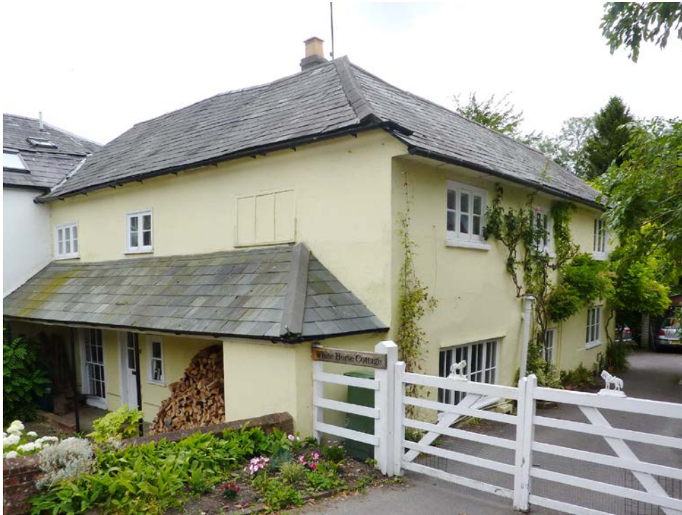
Figure 39: White Horse Cottage , High Street. Now a dwelling but once the White Horse Public House.
