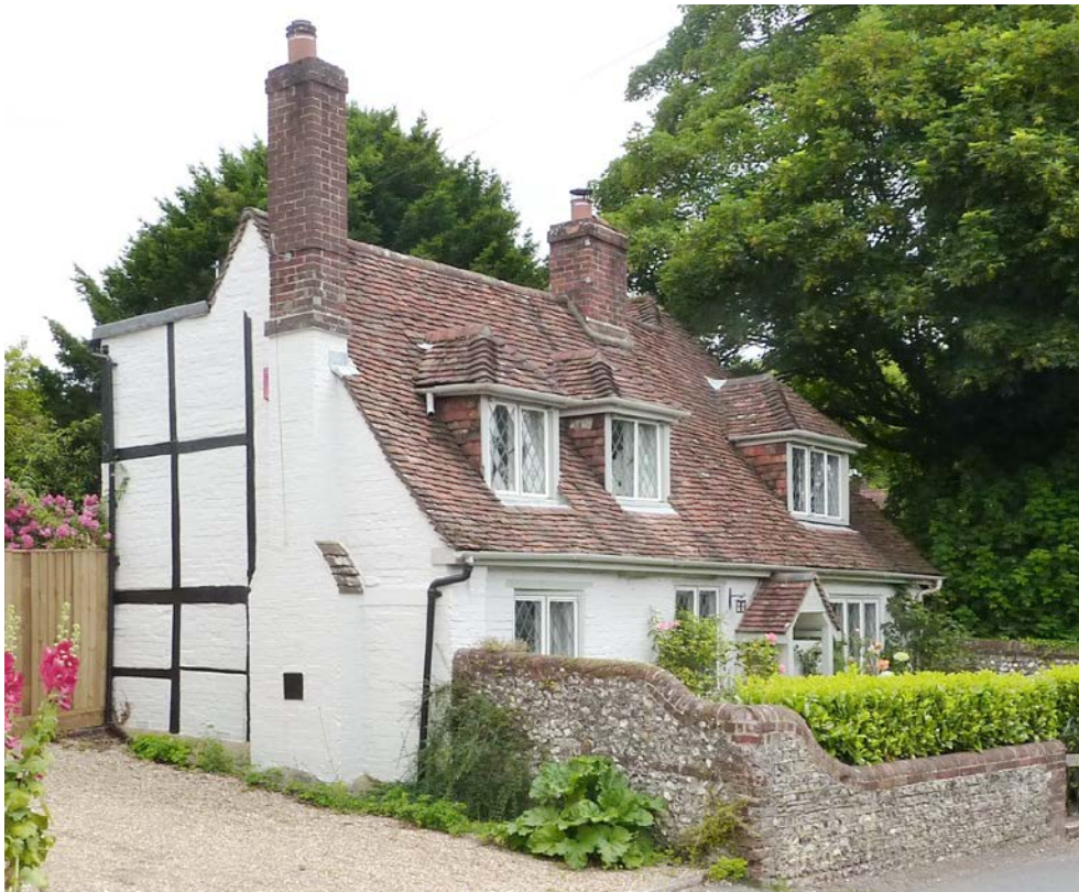
Figure 40: Little Thatch , East Meon Road: A further example of a 17 th century timber- frame with a later brick cladding. Any thatch has long since been replaced by clay tiles.
