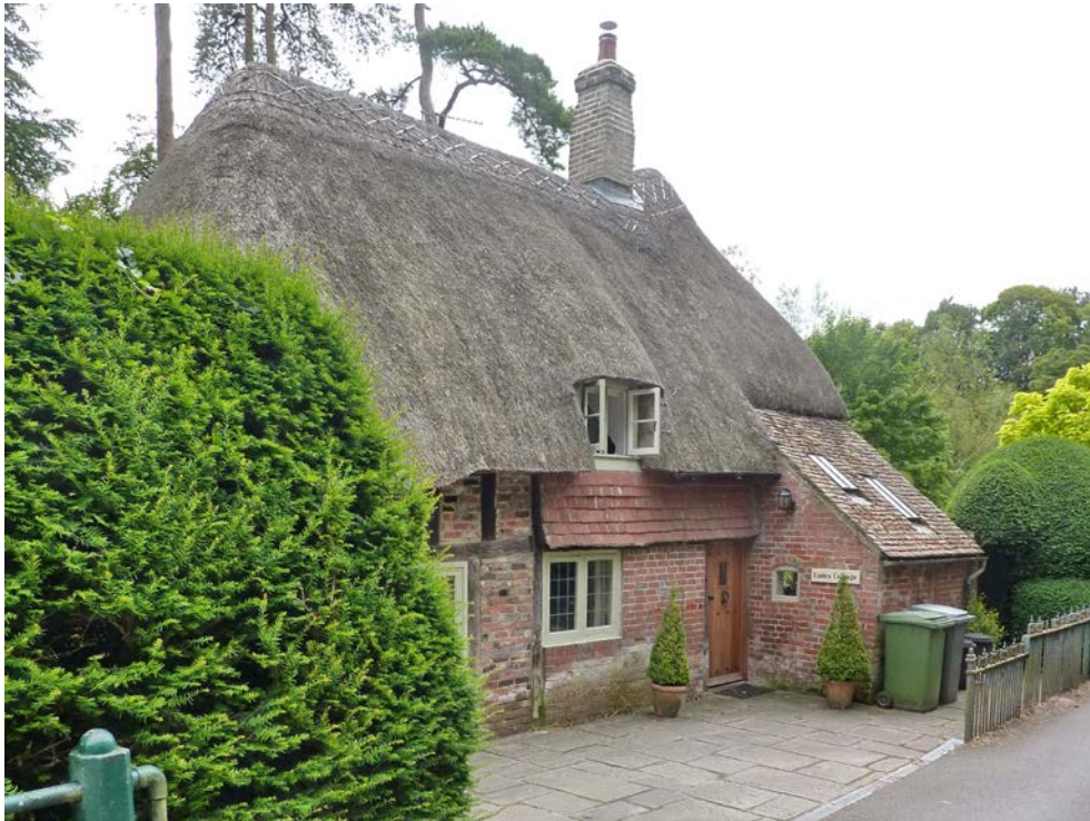
Figure 48: Eades Cottage , East Meon Road. A 17 th century timber-framed cottage sensitively restored in the 20 th century
