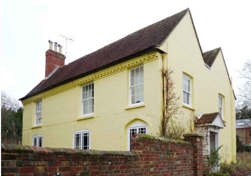
Figure 41: The Grange , East Meon Road. A late 18 th /early 19 th century double-pile house, built of brick in a Flemish bond. The brickwork was later painted.
