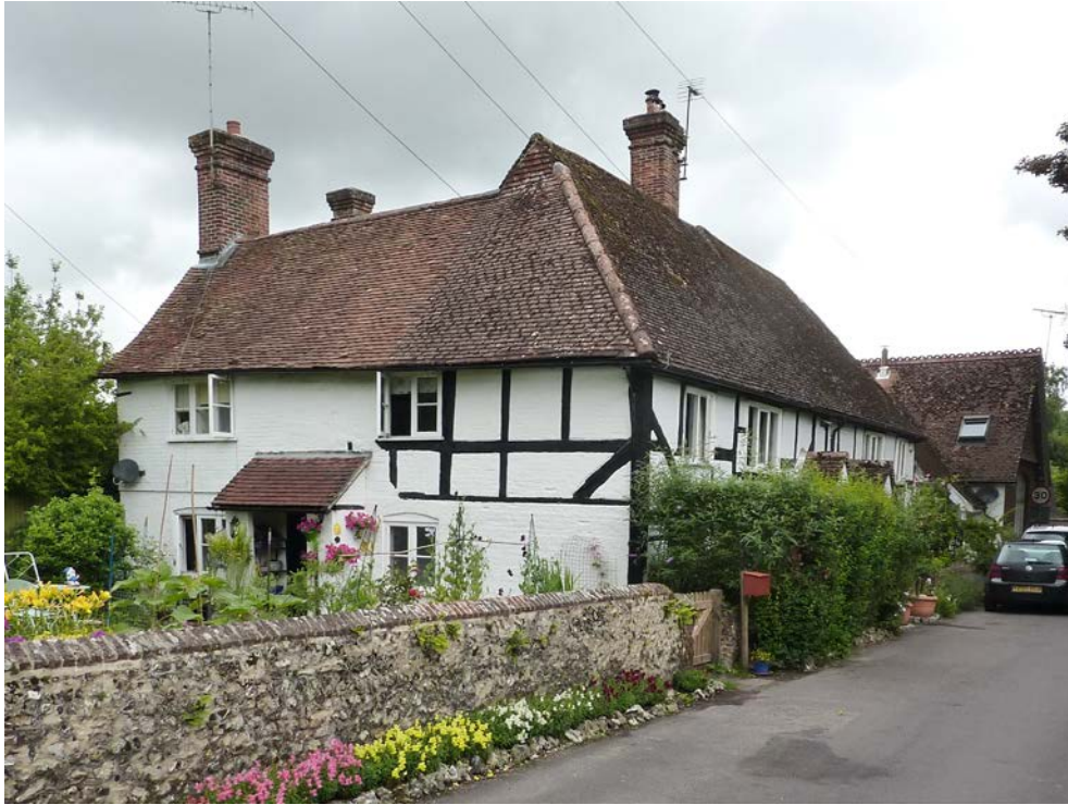
Figure 14: 1, 2 and 3 Station Road. Originally a single dwelling of late 16 th century origin, with 19 th Century rear extensions. The steeply pitched main range was originally thatched.
