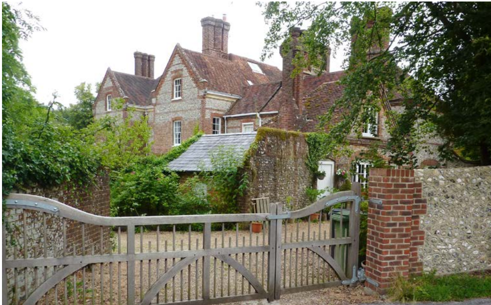
Figure 8: West Meon House and associated service buildings; the house is early 18 th century in origin, with 19 th and 20 th century additions and alterations. Flint is used in the construction of the walls, mixed with malmstone, stone quoining and brickwork to produce a most attractive, mellowed character. The large chimney stacks, Tudor in style, were added in the late 19 th century.
