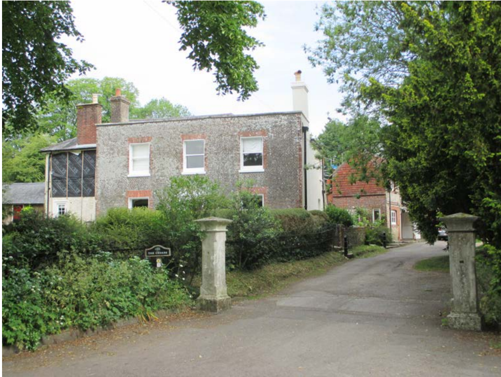
Figure 46: The Cedars , Doctors Lane: early and mid 18 th , with a late 19 th century rear extension. The front wall, which represents a re-fronting of an earlier building, is formed of blue header bricks with red brick dressings, a pattern seen elsewhere in Hampshire but only in this one instance within West Meon.
