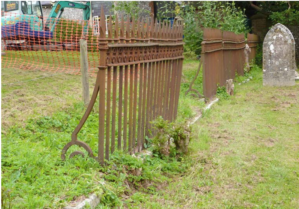
Figure 22: Railings and gates in the churchyard.
