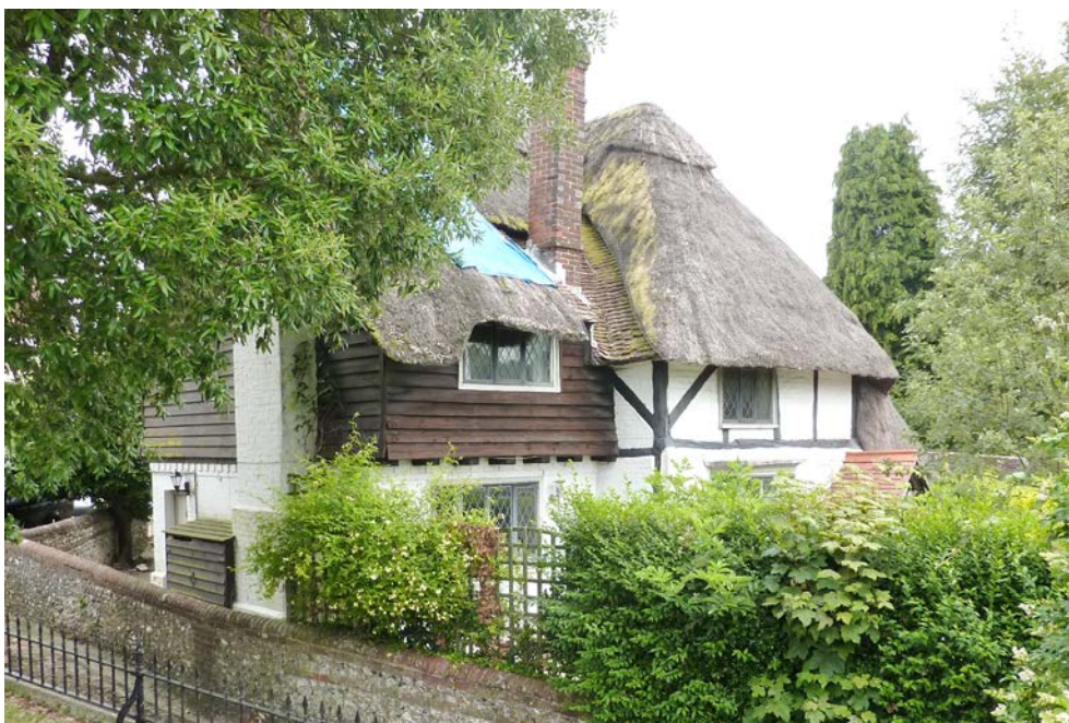
Figure 28: Springfield Cottage , The Cross. Another 17 th century timber-frame with 19 th century brick cladding
