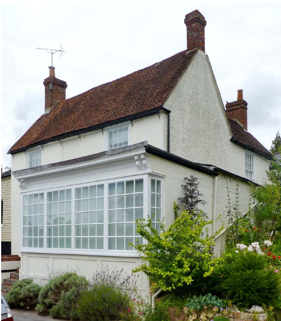
Figure 32: Lassingham House, The Cross, which preserves an early shopfront.
