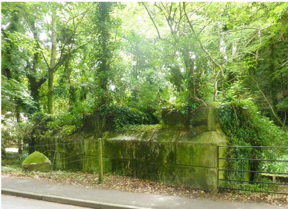
Figure 47: One of the surviving concrete piers from the former railway viaduct. The iron superstructure would have dominated the valley between 1903 and its removal in the 1960s, following closure of the line.
