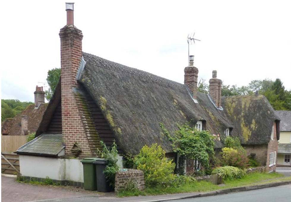
Figure 33 and 34: Cross Road Cottages , The Cross. Another instance of a 17 th century timber frame with later brick cladding, late 18 th century in this instance, although some elements of the frame remain visible. What was once a row of small cottages is now a single dwelling. The thatched roof has a simple, plain ridge detail, which historic photographs show was the usual form in the past.
