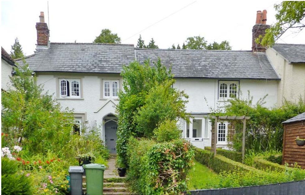
Figure 31: Yew Tree Cottage, The Yews, and Beaconsfield, The Cross.
