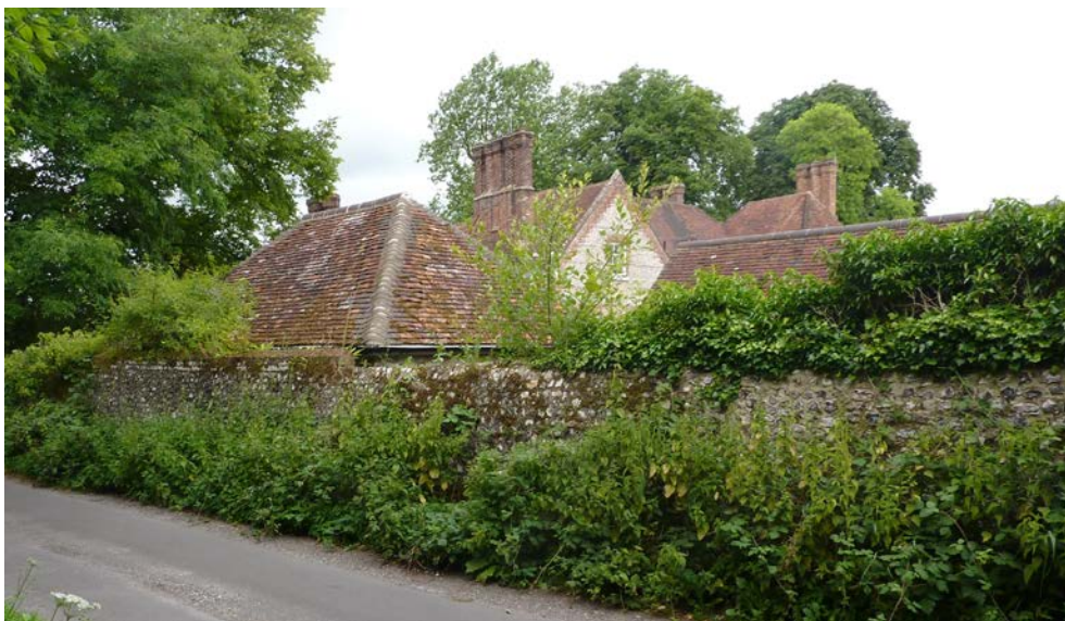
Figure 9: The Service Ranges to the south of the main house and the flint boundary walls also make a significant contribution to the quality of the whole composition.
