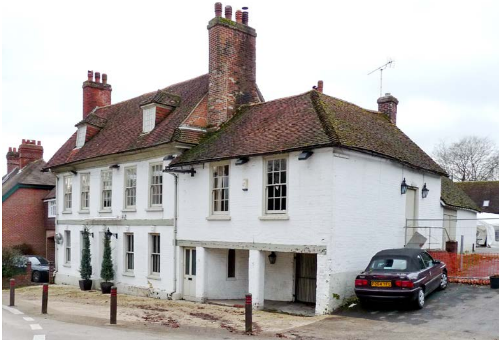
Figure 52: The Red Lion Public House: early 18 th century, with early 19 th century lower wing to the north side.
