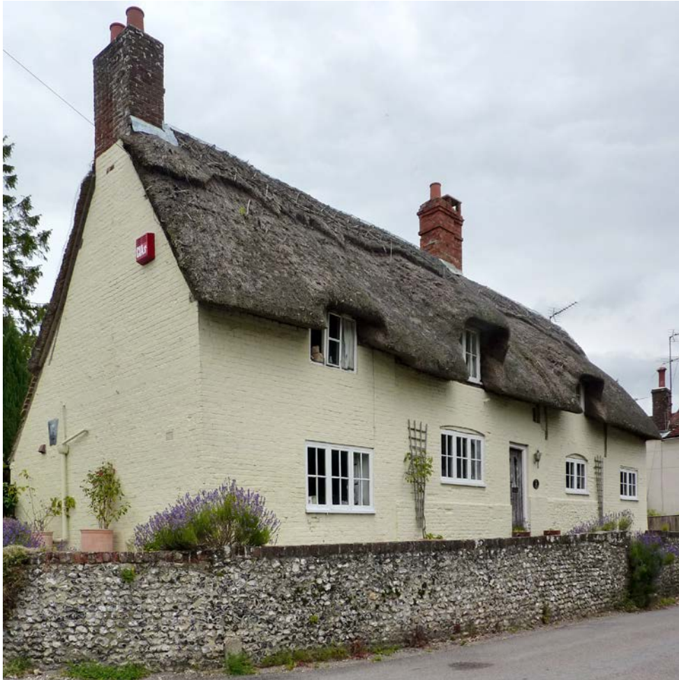
Figure 27: The Cross , at The Cross: Hidden behind the early 19 th century brick cladding is a 17 th century timber-frame.
