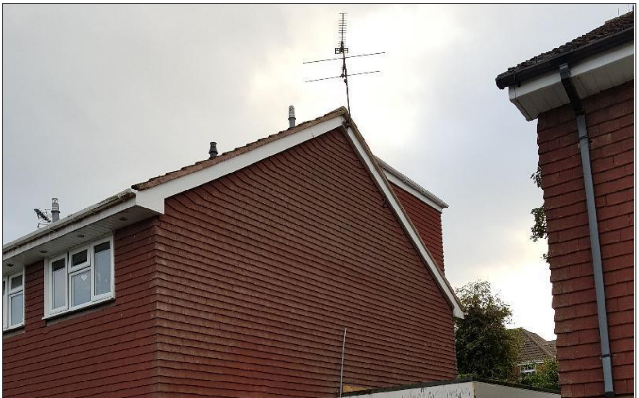
Figure 1 – Dormer Window at 17 Sycamore Drive
