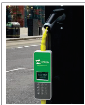
Example of Ovo energy / Ubitricity 3kW lamp post mounted residential slow charger
