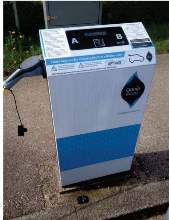
Existing 2 x Chargepoint Genie 7kW unit as installed at South Winchester Park and Ride
