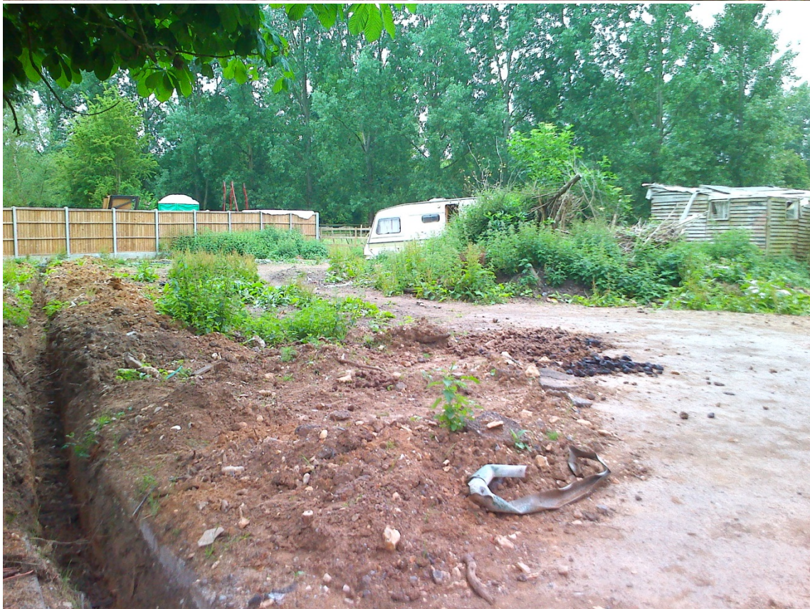
Drainage run – serving plot 3 Unoccupied caravan and looking towards plot 3
