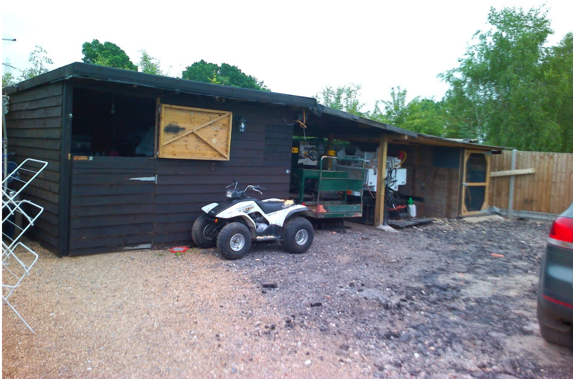
Stables, kennels and equipment shed to the rear of plot 8
