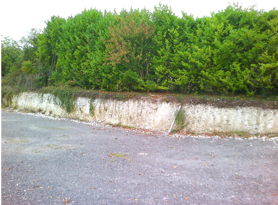
Photo 5 Facing West approx. 2m drop in levels
