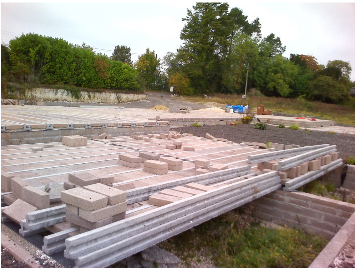
Photo 2 Looking towards entrance from within site
