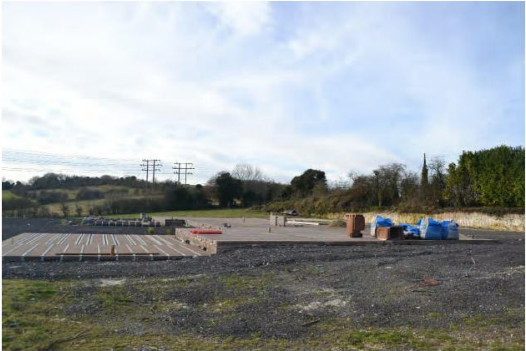
View of works undertaken looking south
