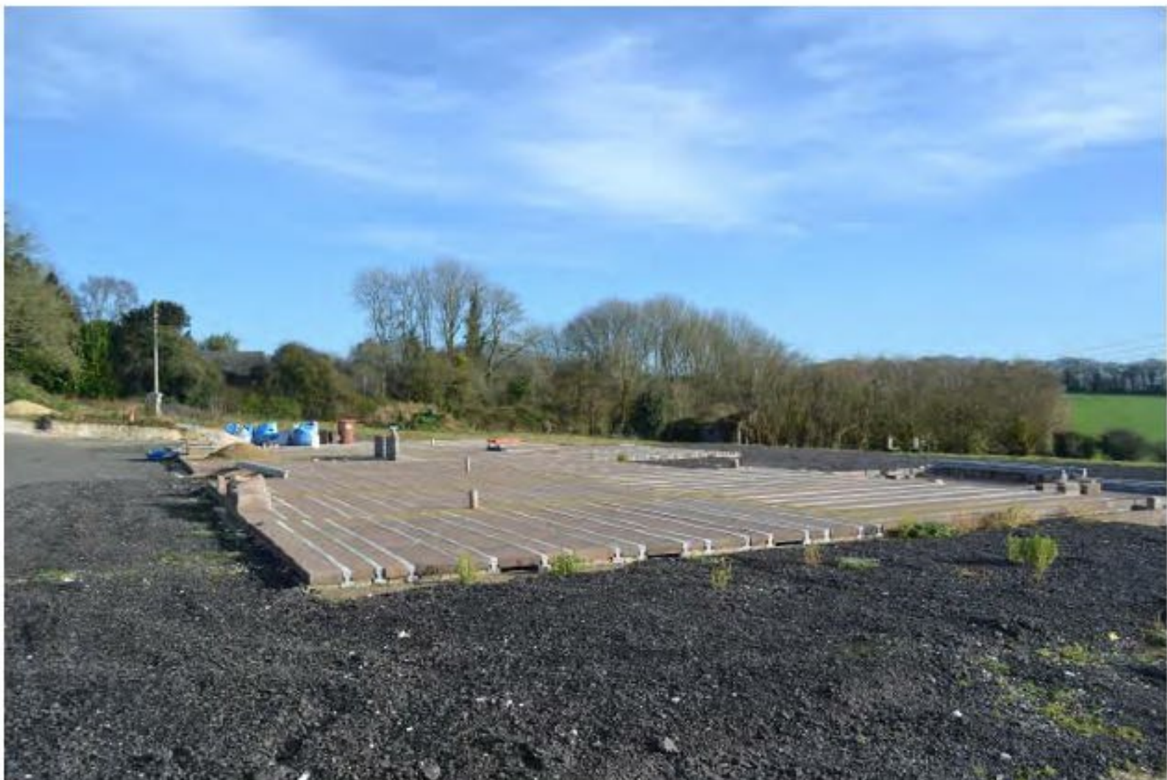
View of works undertaken looking north
