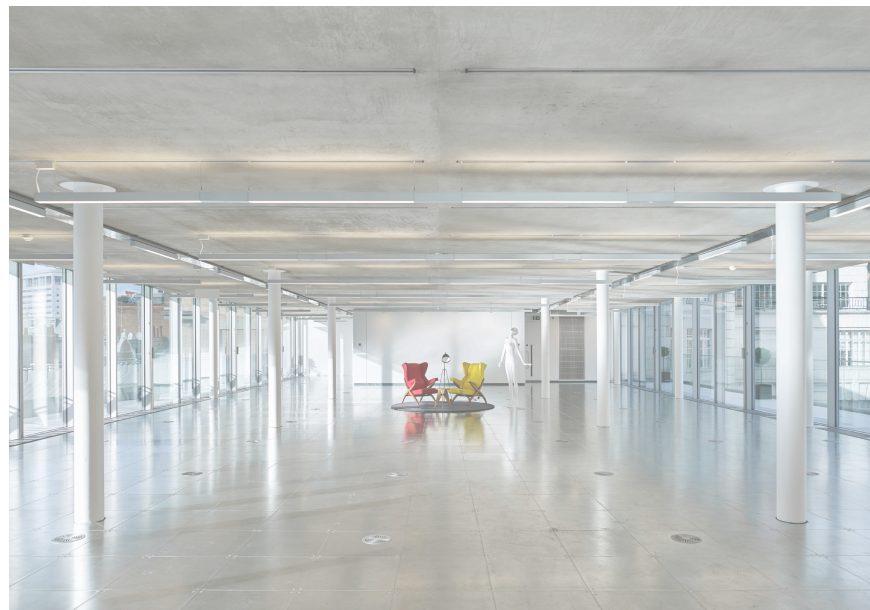
04. Davidson Building, Southampton Street: office space with exposed soffits. Lifschutz Davidson Sandilands
