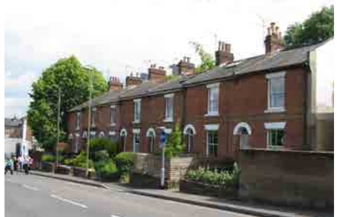
Gladstone Street: Simple terrace in good condition
