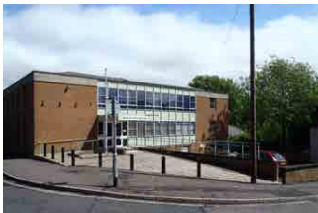
Newburgh House: Low quality building with car parking to front
