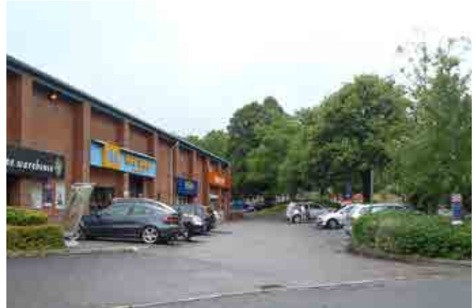
Industrial Style Units: Surface parking facing Andover Road
