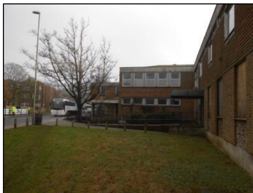
Figure 3: Amenity grassland on the northern elevation of building 1
