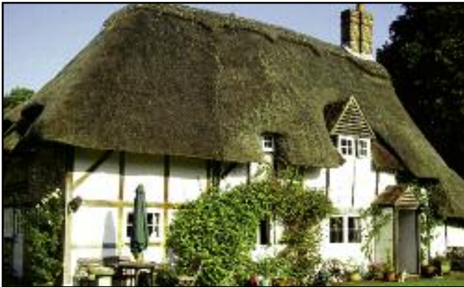
The Homestead Listed Grade II C.17 c.1650 Timber frame, brick infill. Thatched roof. Skilful recent extension at (L) preserves its character.
