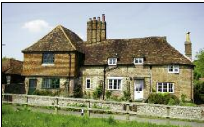
Grove Cottages. Listed Grade II, C.16 (c. 1550) Late medieval Hall house with cross-wings. C.16/17 timber frame, C.18/19 cladding. Probably the oldest/longest lived-in dwelling in Exton. Now 3 dwellings: No 1 (L). Middle (C), Sunnyside (R). 1980 Various extensions to both floors and 2007 other internal alterations. Interesting chimney stack.
