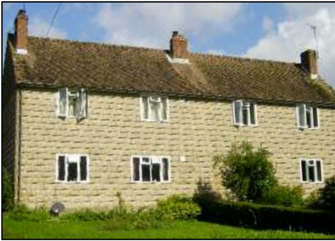
Nos 3 and 4 Larrymore Cottages 1948/9 'Airey' houses, built with pre-fabricated materials by Droxford RDC after WW II to provide temporary accommodation (supposedly 25 years). No. 3 is the only remaining council house in the village.
