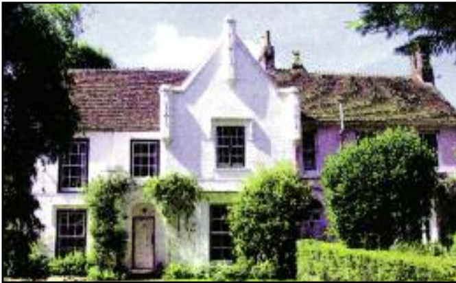
The Old Rectory and Old House Listed Grade II C.18 with early and mid C.19 changes. Walls mostly painted brick, Sash windows. East ('Gothic') wing (L) now The Old Rectory: Porch, pillar and hoodmoulds over three north-facing windows. West ('Victorian') wing now the Old House School-rooms added for Rector's and village children's schoolrooms until proper school (now) Jays Croft built 1871. (See also p.21)
