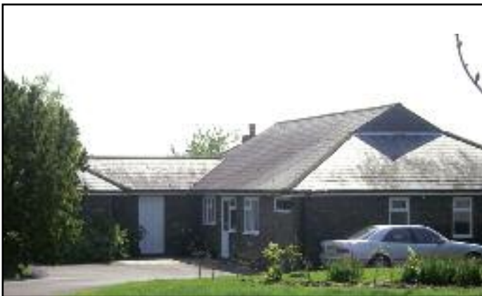
Northcroft Built 1977 on site of wooden bungalow. Being in a poor state this was pulled down and present dwelling built on the same site. Dark brick structure and shallow slate roof are designed to be hardly visible in the AONB SU 608 211
