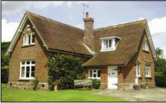
Jays Croft 1871 Built for village School. (Closed 1926). In WW II used as a lay apart store for MTB engines 1952 Converted to bungalow. 1969 Further 1st floor additions with dormer windows. 1992 Conservatory added.
