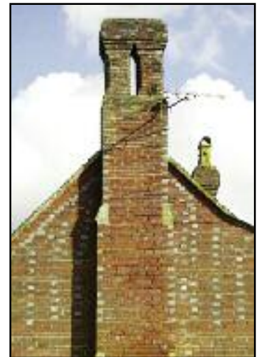
The Old House (W) elevation. Good example of Flemish Bond Also used on Tinnisbourne.
