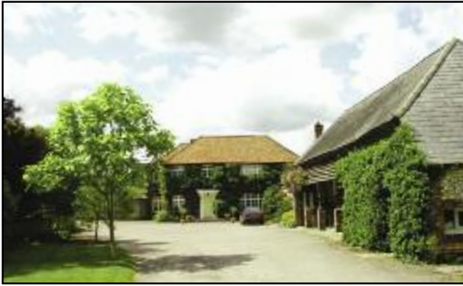
Manor Farm 1964 extension added from derelict farm buildings to provide a private agricultural dwelling.
