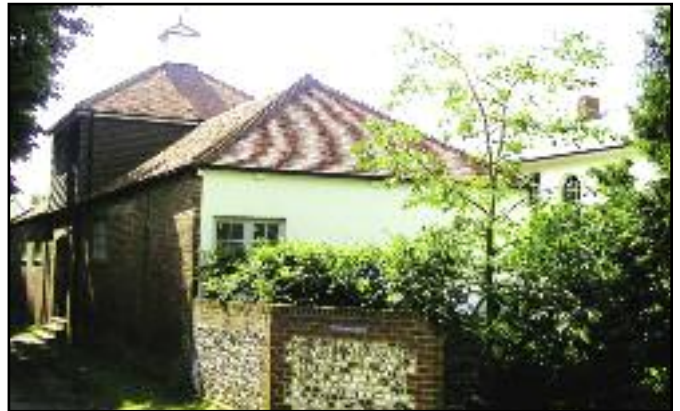
Tinnisbourne Probably late C.19 Part of Exton Cottage estate Converted post WW II from Racing Stables to private dwelling. Recessed porch on lane-side elevation with tiled roof and lantern. Recent extension leading to neo-Georgian wing with slate roof at (R), hardly visible from the Lane.
