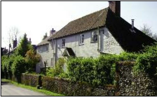
Primrose Cottage Late C.17 for farm worker Extended/rearranged over the years. Note recent extension at (L), subordinate to principal elevation bordering the Lane.
