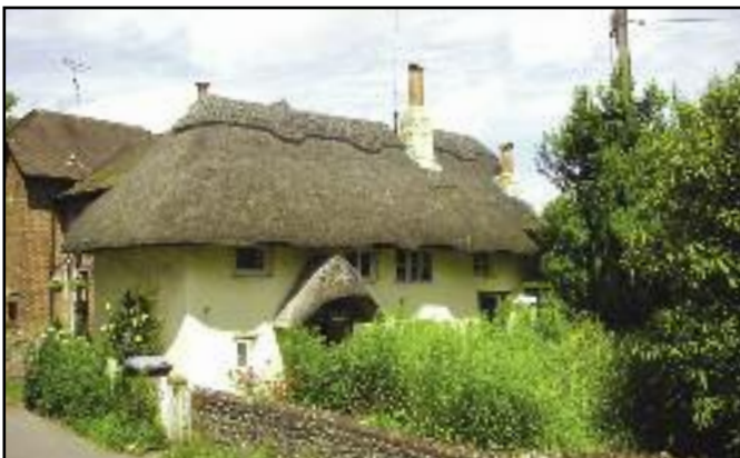
Sunrise Cottage Listed Grade II C.18, early C.19 features. Originally carved out of the chalk bank for a horse and cart, and a smithy for shoeing horses. Thatched roof, rendered cob walls, gabled, boarded porch. Old well in garden. Beacon Cottage behind (L).
