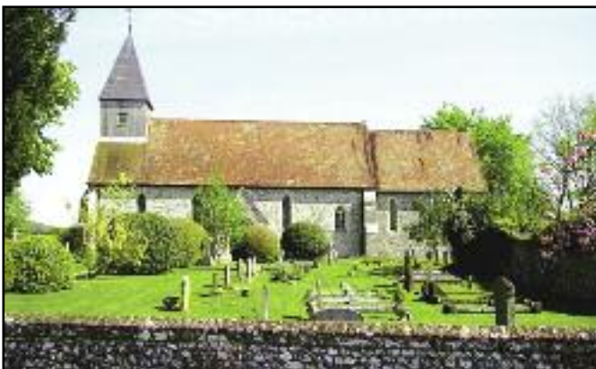
Church of Peter and St Paul . Listed Grade II C13. with masonry evidence from C.15 and C.16. 2-cell Old English structure: stone and flint walling. 1847 and 1892 Much restored and repaired. 1893 Further internal and external alterations. Porch with knapped flints added.
