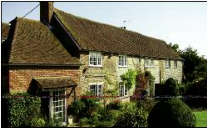
Tithes and Broom Cottage. Listed C.17. Timber frame with early C.19 cladding, and C.20 renovations, including west wing of brick work with a hipped roof. A variety of brick and flint work style. Timber framing exposed within. Once a Barn now two dwellings in a single range: Tithes (L), Broom Cottage beyond flint wall (R).
