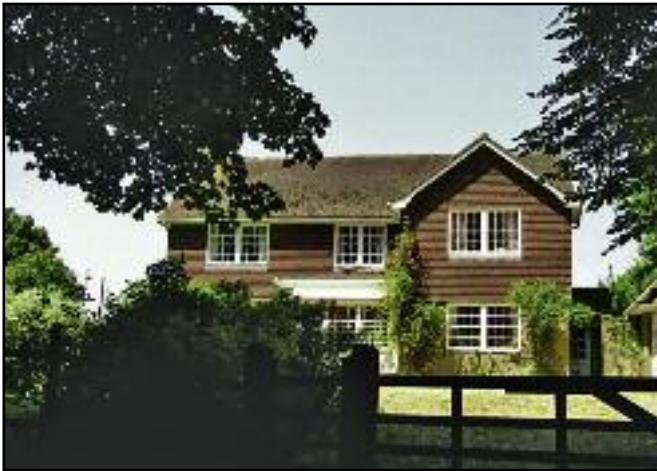
Bramcote House 1976/7 Purpose built private dwelling with part tile hung elevations Designed and constructed by first owner Approved by Winchester CC.
