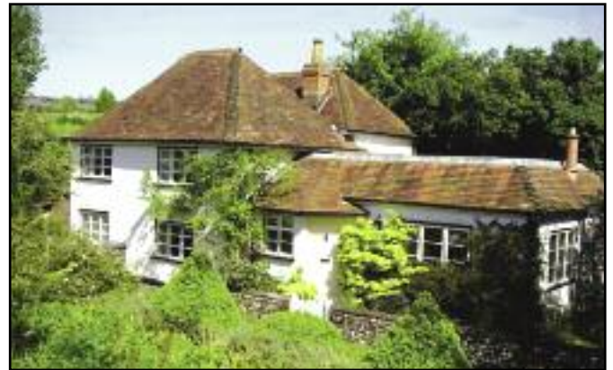
Wild Rose Cottage C.17. Former Farmworker's cottage. Painted brick structure, Tiled roof. Part timber framed, part painted flint, part rendered 'cob'. Part painted brick elevations. Tiled roof. 1997/8 Major porch and 1st Floor extension at rear 1992 2nd Extension single storey at rear.
