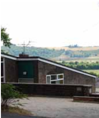
HOUSING SET INTO THE SLOPE ALLOWS PANORAMIC VIEWS OVER ROOFS
