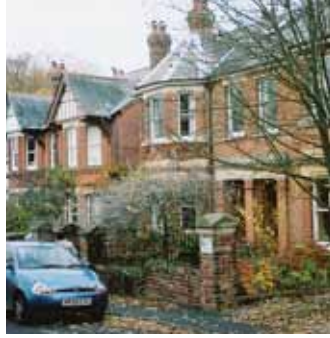
OLDER SEMI DETACHED PROPERTIES SET BACK FROM THE ROAD WITH ROOM FOR SHRUBS AND TREES
