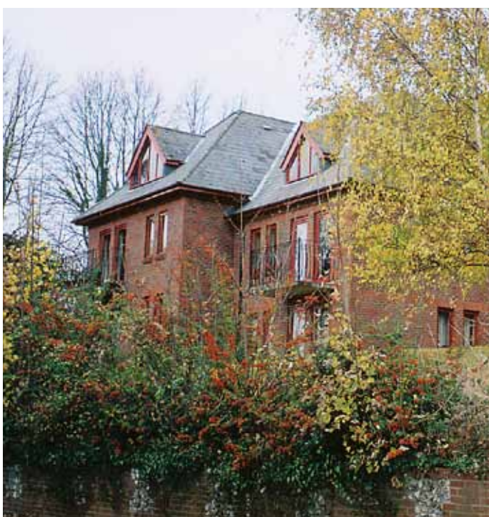
3 STOREY FLATS WITH BROKEN ROOF LINES AND TREE COVER
