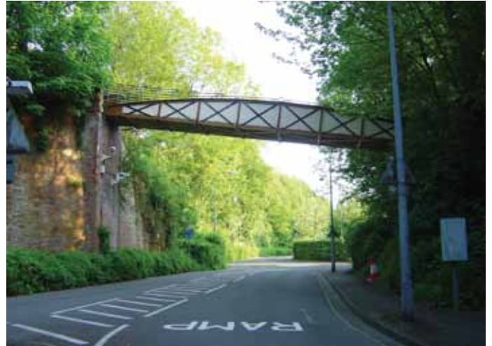
THE RESTORED RAILWAY FOOTBRIDGE
