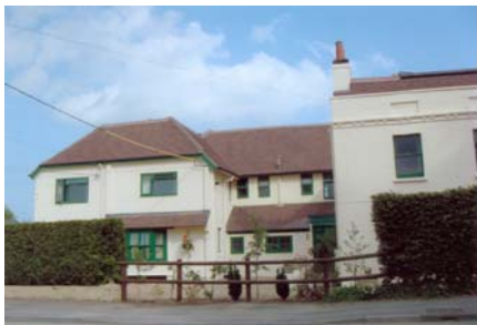
Elderfield before and after renovation
