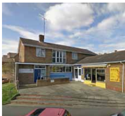
Former Library site
