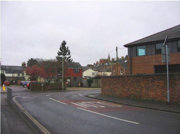
Figure 28: Prominent corner on the tight bend on Gordon Road
