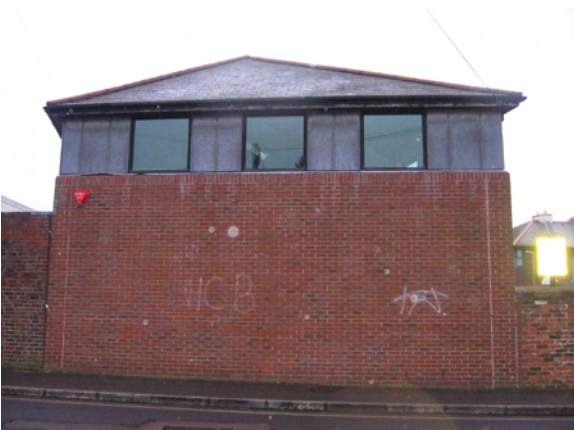
Figure 29: Blank frontage on the southern side of Gordon Road
