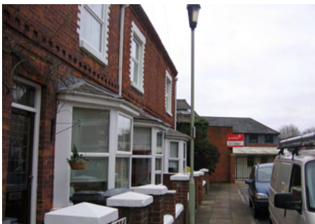
Figure 5: View looking east along Hyde Abbey Road to the site
