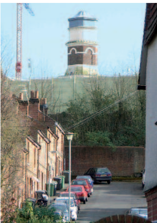
View to Greenhill Avenue and the prison
