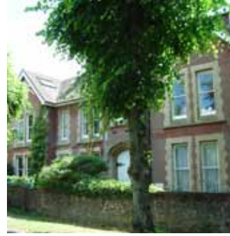
OLDER PROPERTY CONVERTED TO FIVE DWELLINGS
