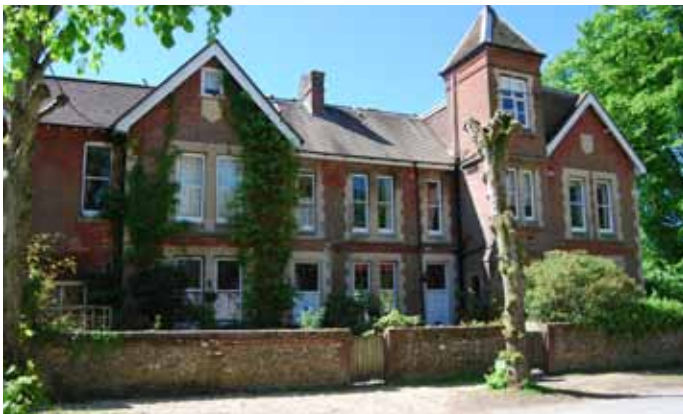
OLDER 3 STOREY PROPERTY CONVERTED INTO FIVE DWELLINGS
