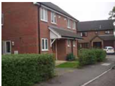
Modern housing at Meadowcroft Close
