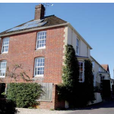
Mill House – red brick and render
