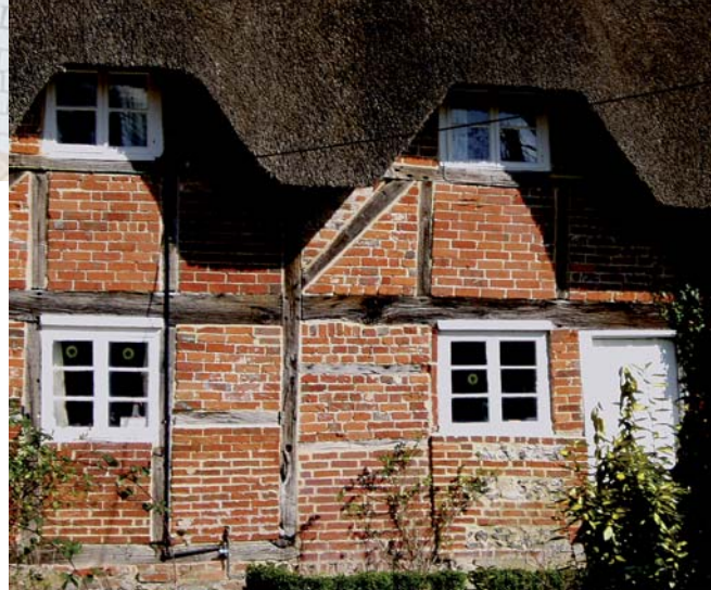
6 & 7 Mill Lane timber frame with brick infill
