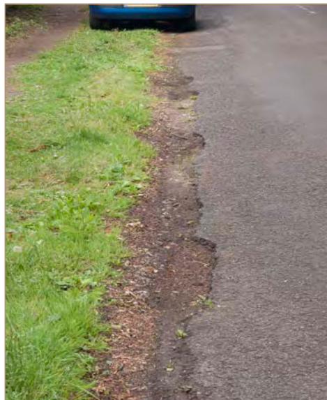
Damaged road edge
