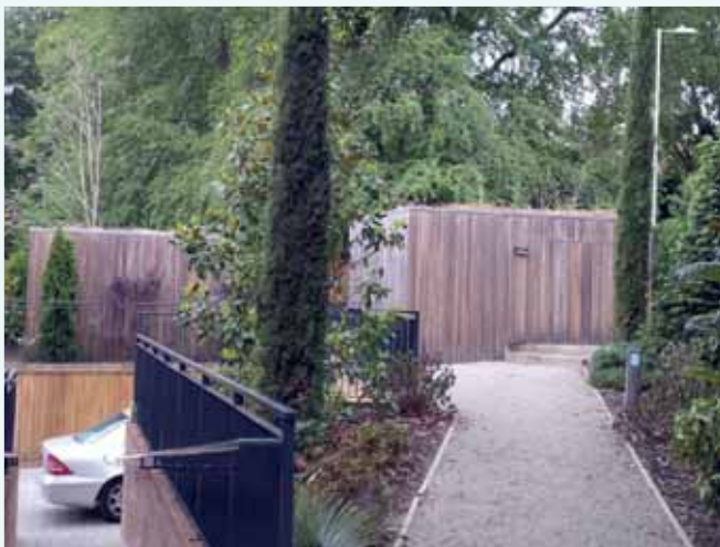
Well designed bin and cycle storage at the former Ambulance Station site, Winchester.
