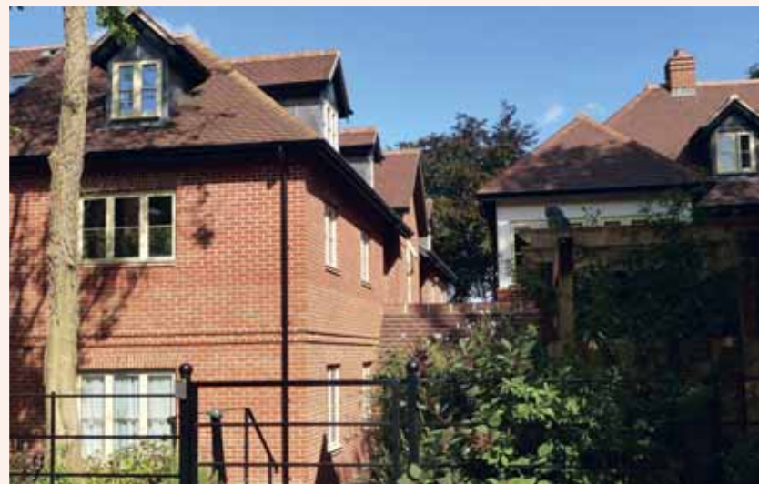
These dormers on the Milesdown development in Winchester are elegantly proportioned and well related to the rest of the fenestration. The materials and detailing are high quality.
