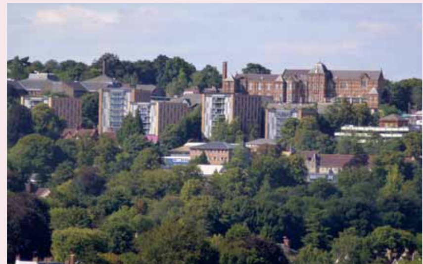
This example of high quality new development at Winchester University illustrates the impact of topography, and also the need to consider the impact of new buildings when seen in long views.
