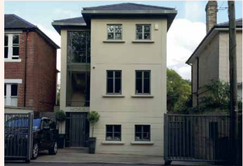
The proportions of the front elevation are slender and elegant. The arrangement of windows using different sizes in an ordered way, reinforce that impression.
