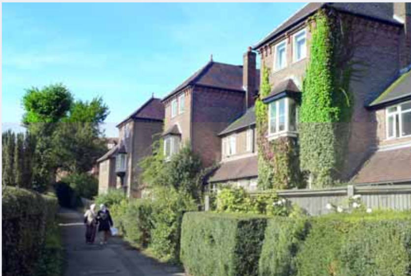
The quality of this footpath in Hyde is enhanced by the height and design of the buildings, which provide enclosure and surveillance.
