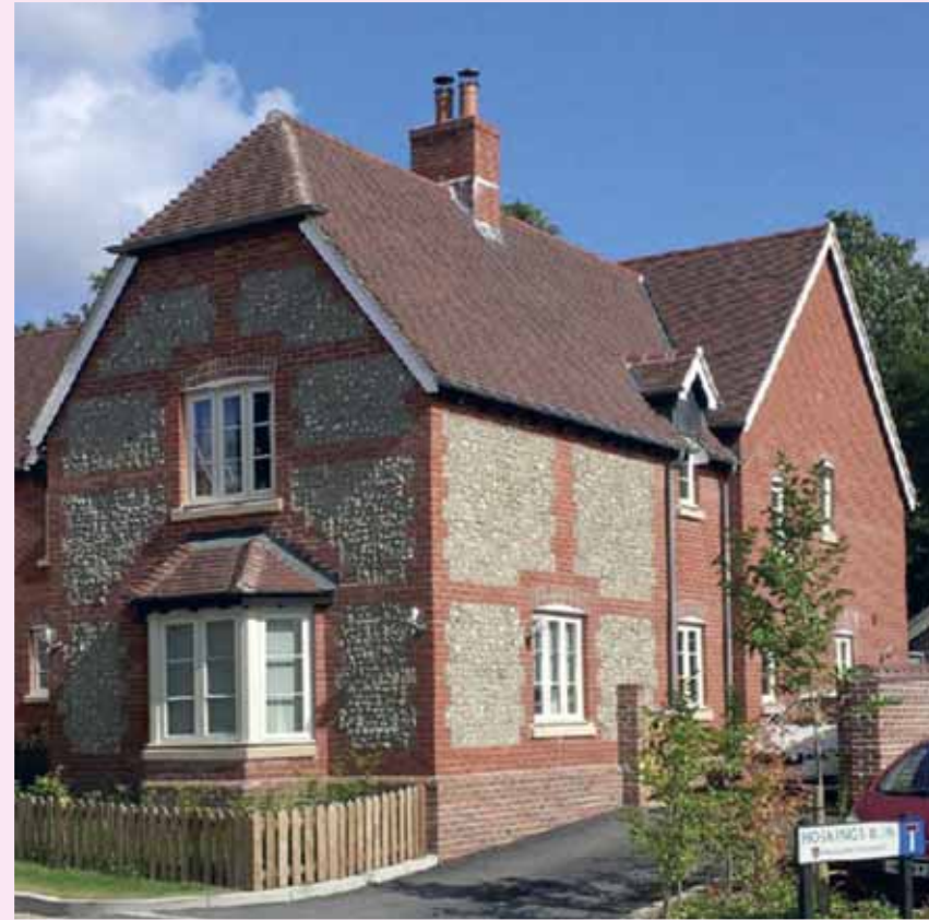
This flint walling in Cheriton is successful, giving a textured, traditional appearance. The brick quoins also play a significant role in the success of the finish achieved.
