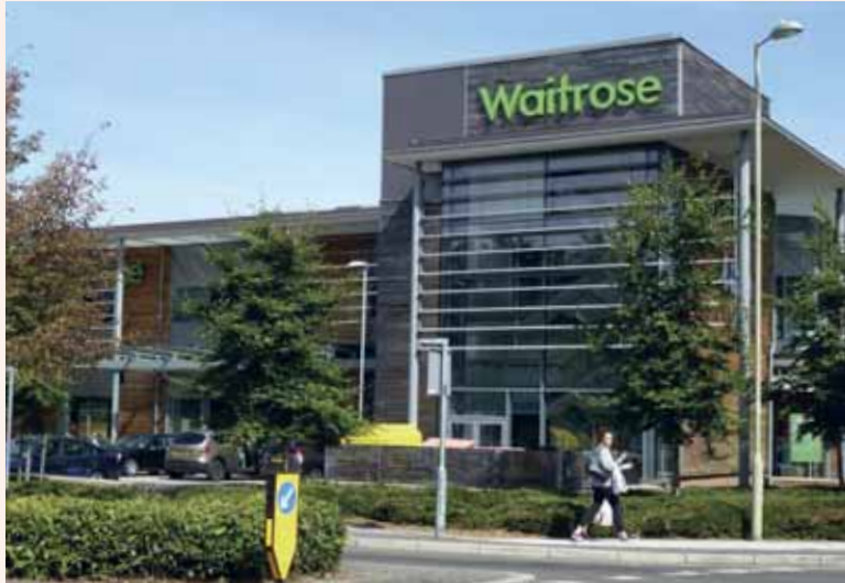
This example in Weeke in Winchester is a good example of where built form has been used to emphasise a corner to draw attention to what is an important local centre.
