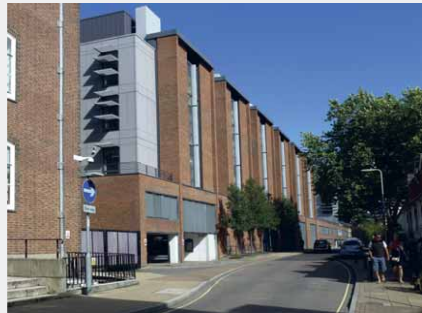
The new Hampshire County Council offices successfully fit into the street scene by using high quality materials and detailing and a strong sense of rhythm.
