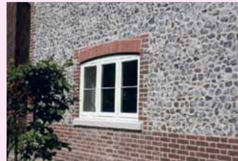
This flint walling in Cheriton is successful, giving a textured, traditional appearance. The brick quoins also play a significant role in the success of the finish achieved.
