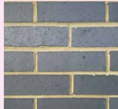
In this example, the lack of colour matched mortar perhaps undermines the appearance of the dark bricks, and the combination with red brick is also not as successful.
