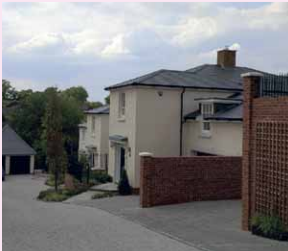
This example on Chilbolton Avenue utilises high quality paviers with subtle differences between the textures and colours creating a successful overall composition.
