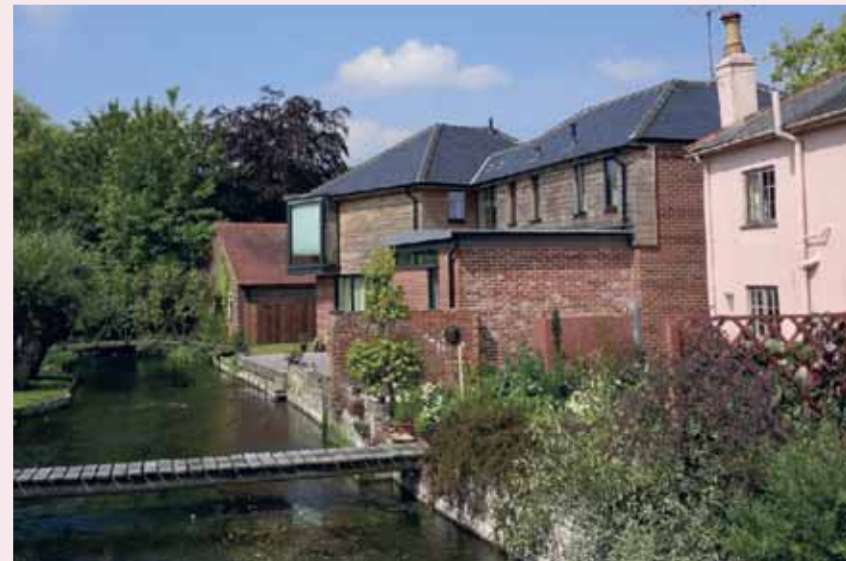
This design in Exton utilises the river to create a very exciting design solution.
