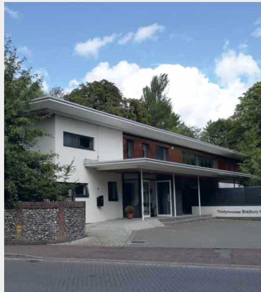
A crisp contemporary design at Durngate, Winchester.
