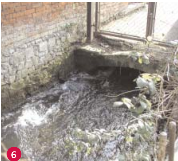
6 Culvert at Buskets Lane
