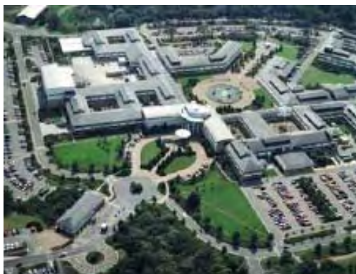
Cody Business Park, Farnborough
