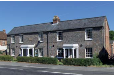
Setbacks of approx 3m of house frontage from back of footpath, Kingsclere.
