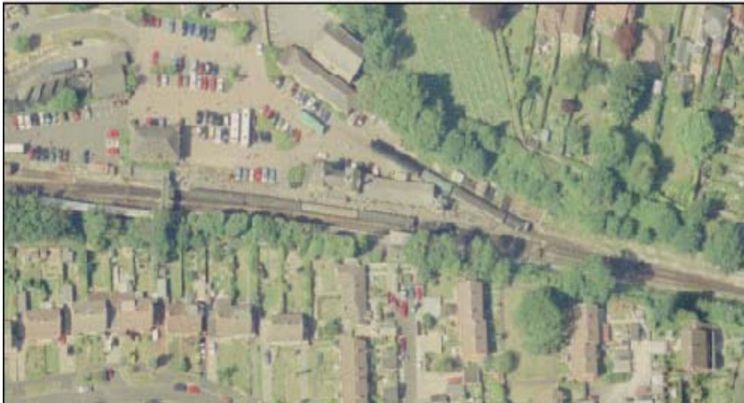
Figure 1 – Aerial Photograph of Alresford Railway Station
