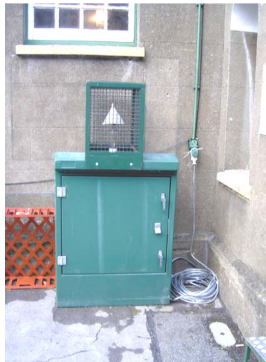
Figure 4 - Cabinet used for second round of monitoring
