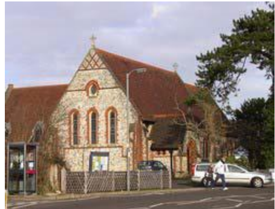
The village church showing the knapped flint and brick quoin construction typical of many of the older buildings.
