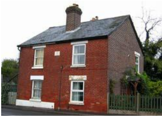
Lynden Cottage of the 19 th century. Brick with slate roof, and sash windows.
