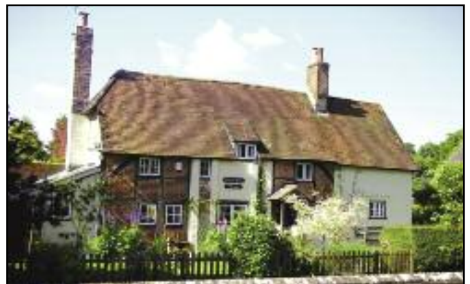
Church View Cottage. Listed Grade II C.16. Tall chimneys indicate cottage was once thatched. Originally two dwellings. Timber framed with exposed brick infill. Covered well. 1947 Painted Brick and tiled roof extension at (R). 1984 Converted to single dwelling.
