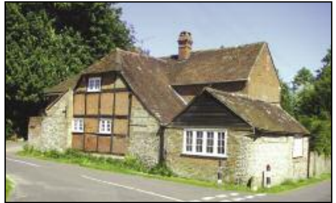
Corner Cottage C.17 De-listed 1972 Part timber frame, brick in-fill Various brick and flint walling Covered well (See p.21) Former tied farm worker's cottage, then a sweet shop 1973 De-listed Grade II modernised and insulated. 2002 Ground and 1st floor extensions.
