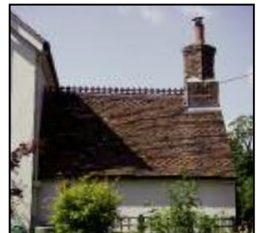
Riversdale - Interesting patterned tiling, for the Headmaster's house. Also on Jays Croft - the former school.
