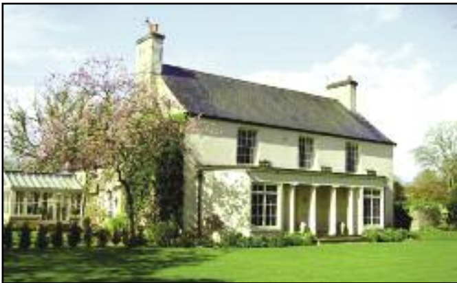
Manor House. Listed Grade II C.17/18 with brick infill, part exposed and part painted. L-shaped plan. South wing C.17 Red brick structure, tiled roof. North wing C.18 Stuccoed brick facade with slate roof, Recessed porch with four columns. 2007 Conservatory added. Mostly sash windows.
