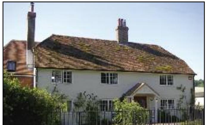
From Allens Farm Lane Allen's Farm. Former farm cottage C.17 Tall chimneys indicate cottage was once thatched. Later additions and alterations 1872 Named Exton House (OS) 1908 Named Allen's Farm (OS) 1998/9 Major renovations SU 607 207
