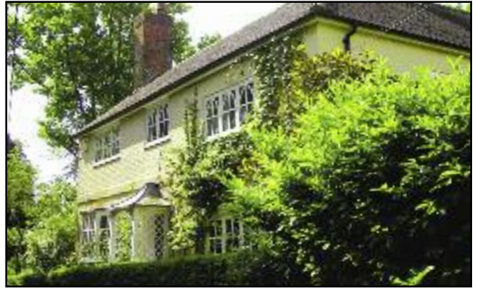
Dairy Cottage Early C.18 designed for cool storage of dairy products. 1979 De-listed Grade II following major restoration: faced with brick and modernised within. 1996 Single storey extension for rearranged kitchen. Porch canopy added.
