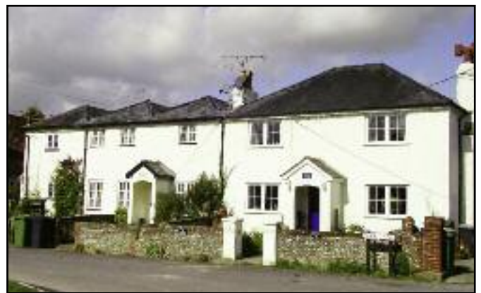
Originally 2 cottages, Wyndham 1 & 2, pre 1839. Named after Mrs Wyndham-Long of Corhampton House. c.1850 Rose Cottage (L) built on to Wyndham 2. 2007 Wyndham 1 (R) Wyndham 2 completely demolished then rebuilt as Kingfisher Cottage (M).
