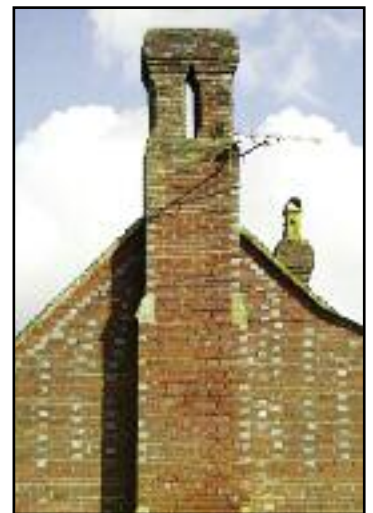
The Old House (W) elevation. Good example of Flemish Bond Also used on Tinnisbourne.
