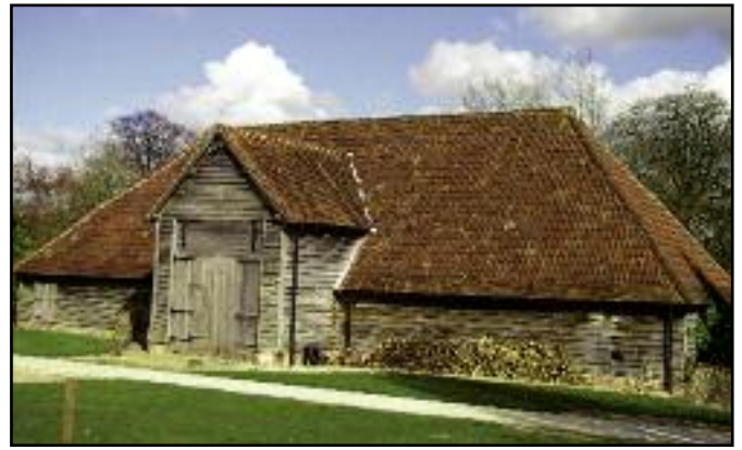
Timber frame, 5-Bay Barn Listed Grade II C.16 with later revisions. Projecting central waggon entrance. Hipped pantile roof, tiles over entrance.
