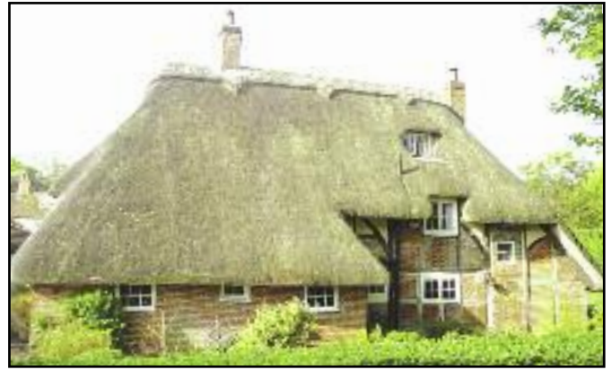
Marriners Listed Grade II C.16 3-bay timber frame exposed with various brick infill. Thatched roof. Covered well. 1984 Modernised within. 1987 Garden room/conservatory added.
