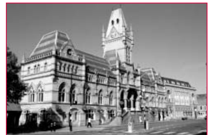
Winchester Guildhall, one of the city's historic buildings, maintained by the Corporate Property Team.
